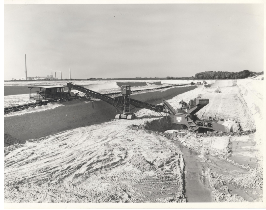
Excavator in Operation
