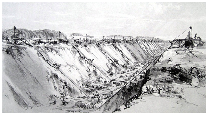
Construction of Tring Cutting, 1837 (Source: GM)
